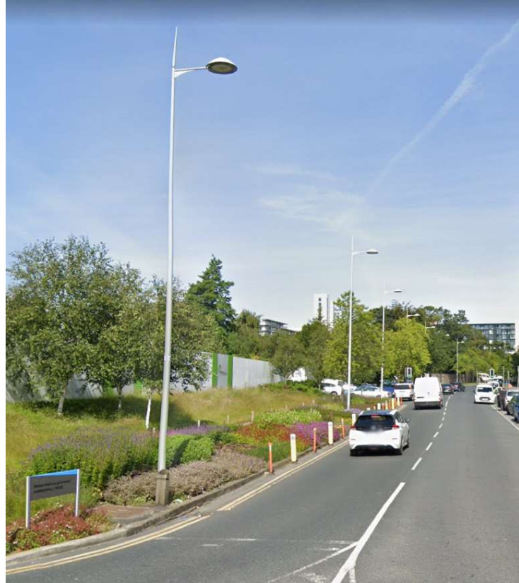
Fig 6.2 Existing DLRCOCO Public Lighting columns on Carmanhall road
